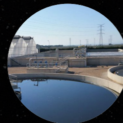
WATER TREATMENT & MINING
